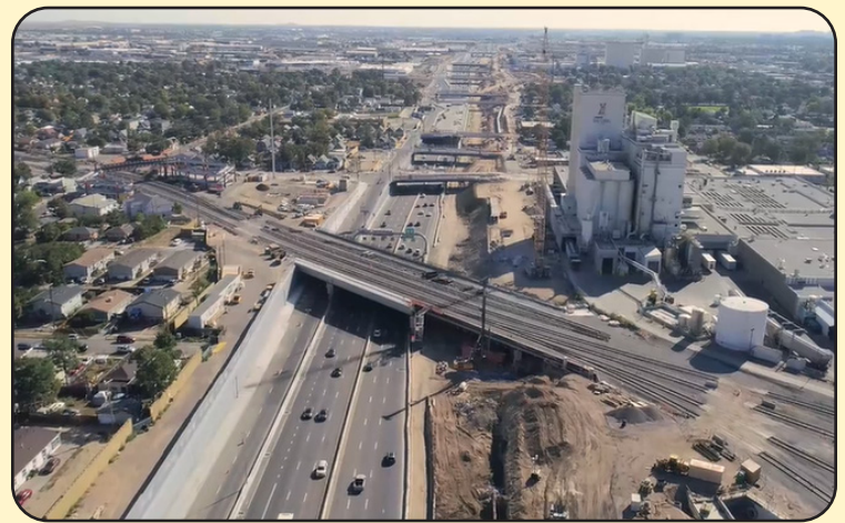
Image 4. Central 70 After Demolition of the Viaduct
