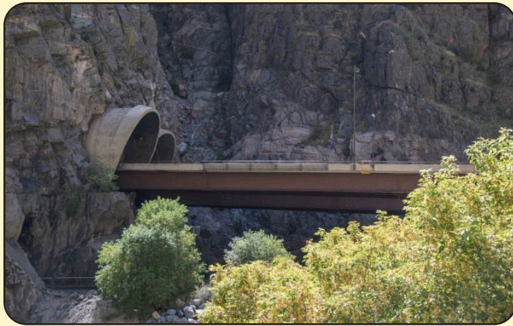
Image 1. Hanging Lake Tunnels (Region 3)
