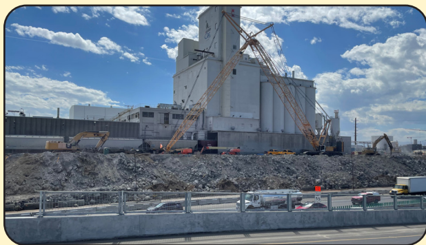
Image 13. Demolition of the I-70 Viaduct at Union Pacific Railroad
