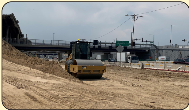
Image 12. Excavation Work of the Future Eastbound lanes of I-70
