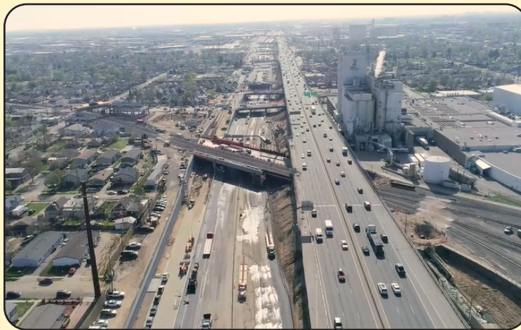
Image 3. Central 70 Before Demolition of the Viaduct
