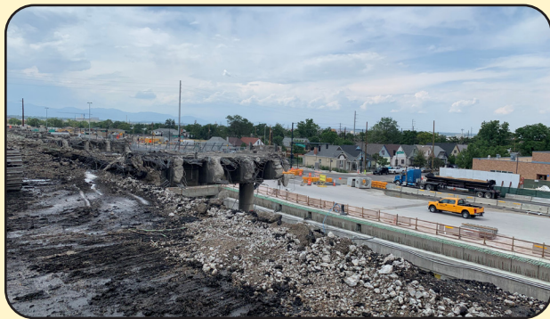
Image 11. Demolition of the Viaduct
