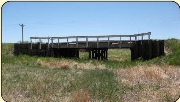
Image 15. I-70 Service RD over Draw in Arapahoe County (F-20-L)
